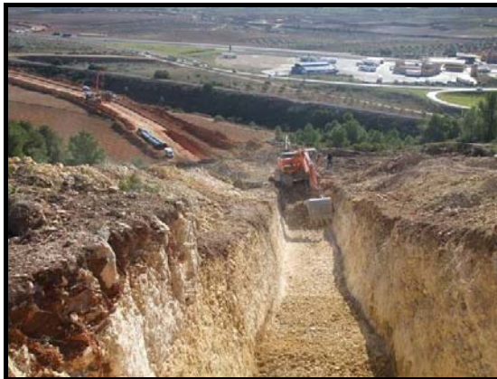
Photo 1: Excavation trench in ascent to Ramblar
