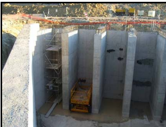
Photo 3: Container housing dumping equipment
